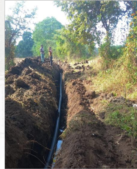
Kishanpura, Madhya Pradesh
